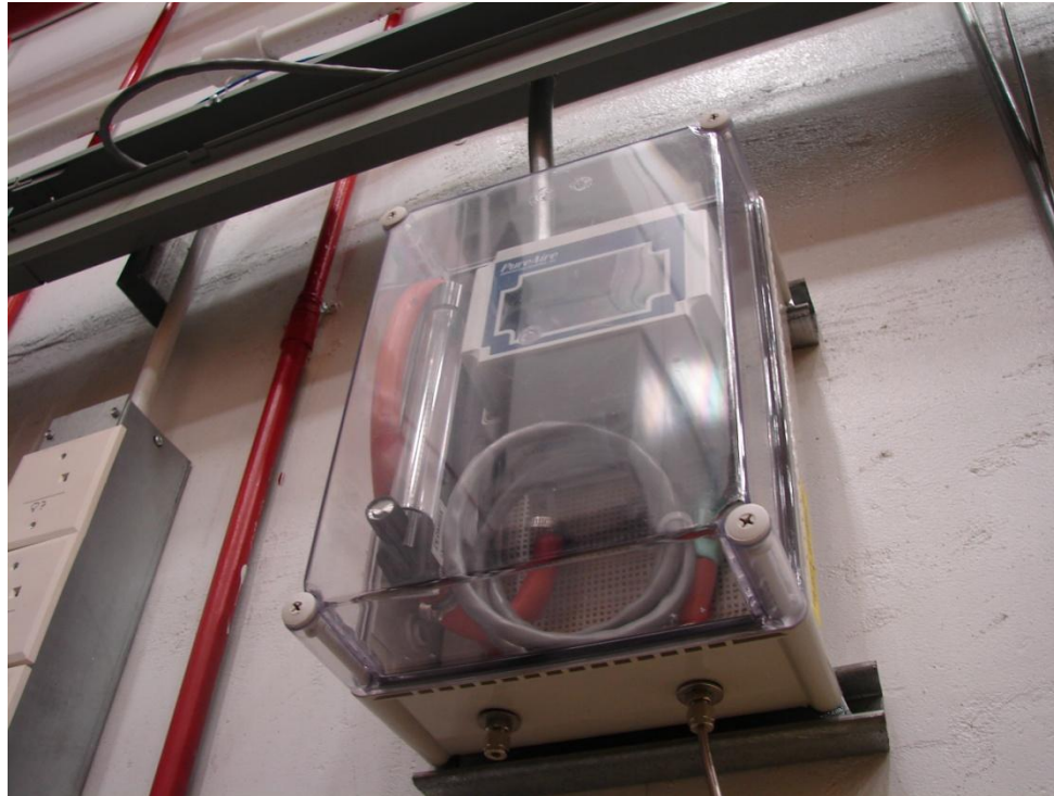
Figure 3 Hall D ODH Sampling Monitor
